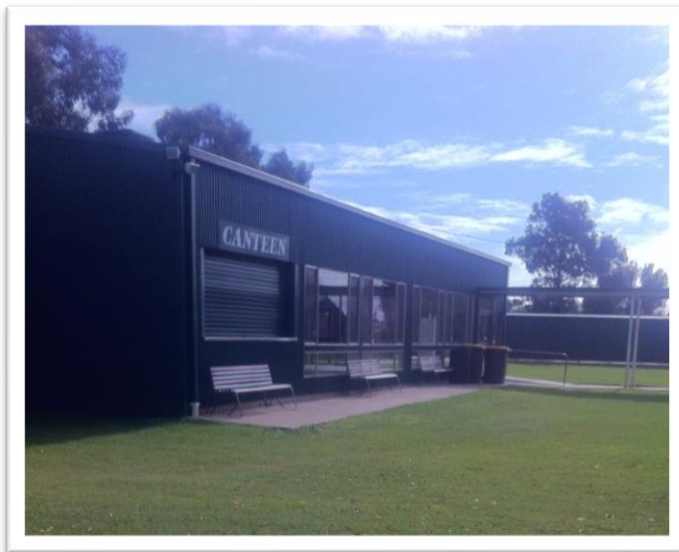
Bar Room and Canteen
