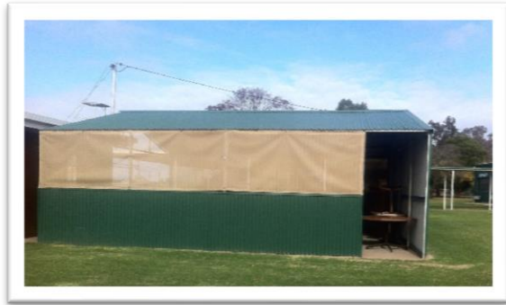
Awning Shelter exterior
