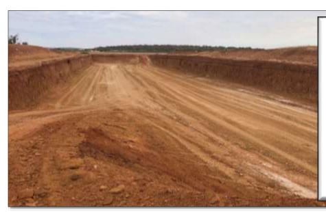
Construction of a new landfill trench (pictured) was completed in June. The leachate pipe system was also connected and the new Leachate pond constructed and has passed the relevant compaction tests. The final stage of Capping the Landfill trenches was also completed with Council using its own Green waste chippings as the final layer of mulch.
