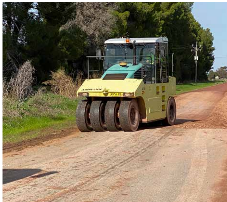
The multiwheel compactor being used on Wagrahm Road
