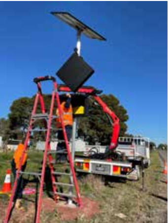
Vehicle Activated Signage being installed at Research Road, Yanco
