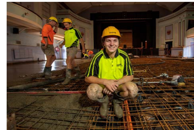
Liam Horton working on Roxy Redevelopment
