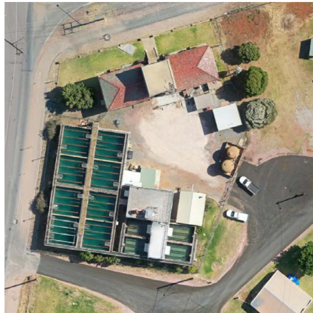
Leeton Water Filtration Plant
