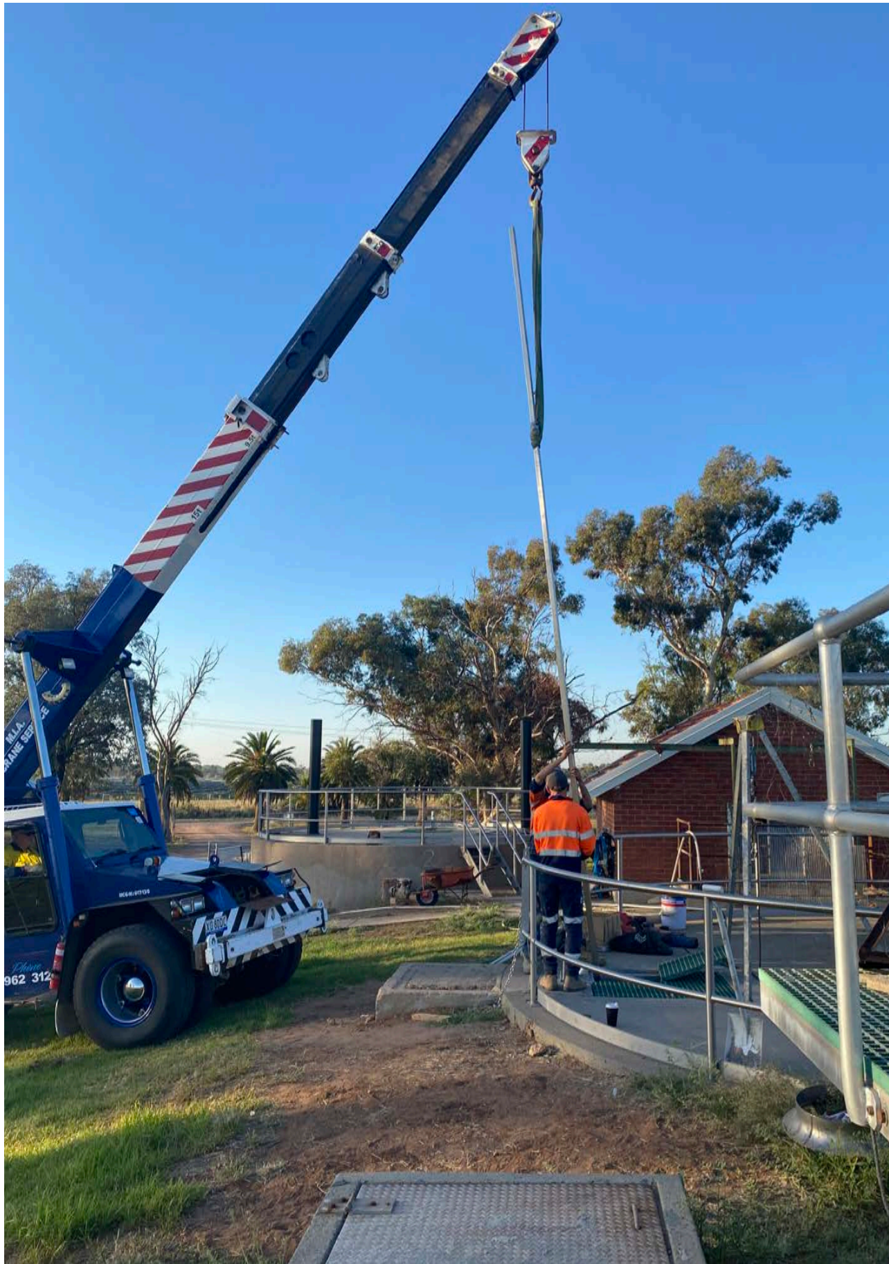
Leeton Sewer Treatment Plant upgrade
