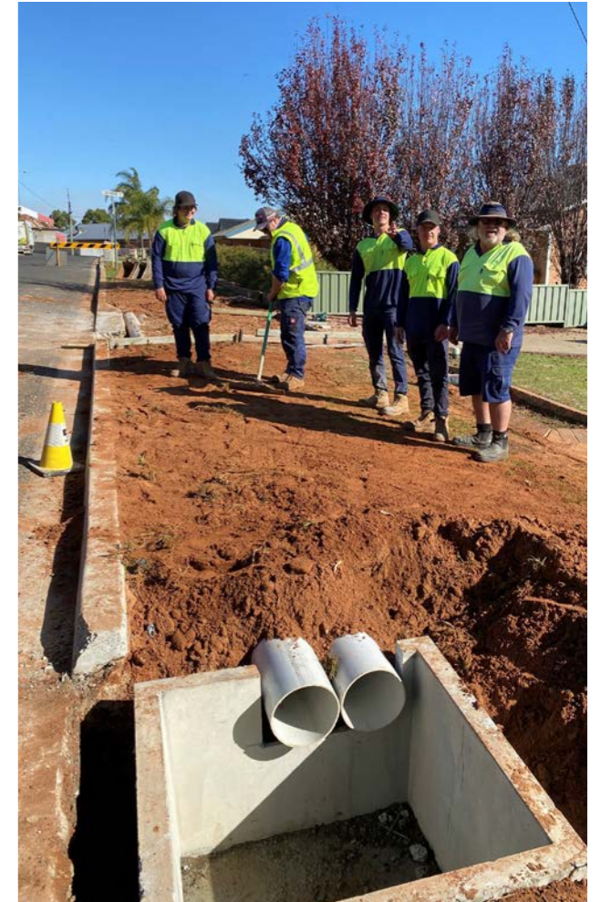
Extending stormwater drainage – Cedar Street
