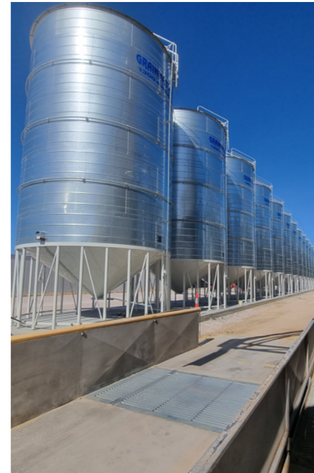
Silo complex at the Voyager Malthouse, certified and signed off by the Certification Team
