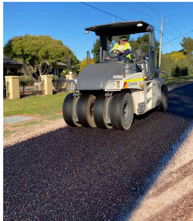
Road sealing works on Almond Road
