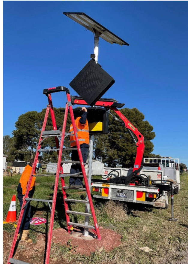
Vehicle Activated Signage installed on Research Road
