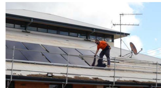
Solar panel installation at the Leeton Shire Library. Installation completed by Ben Walsh Solar and Electrical
