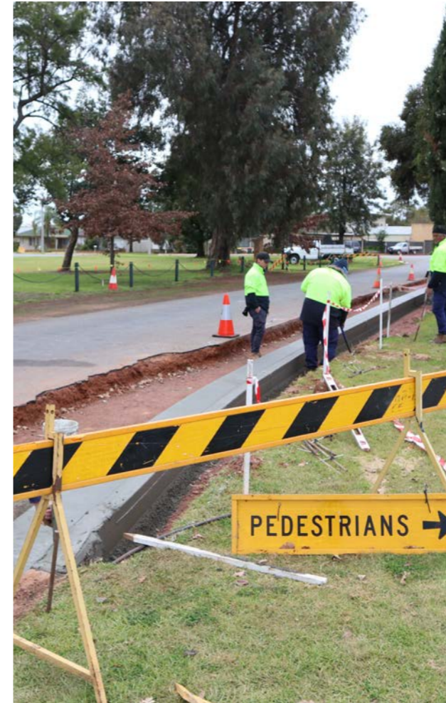
Kerb and guttering Melaleuca Avenue
