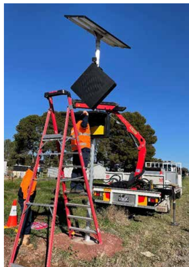
Vehicle Activated Signage installed on Research Road
