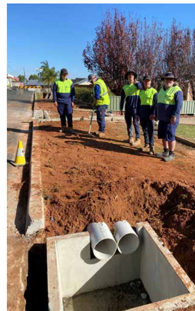
Extending stormwater drainage – Cedar Street
