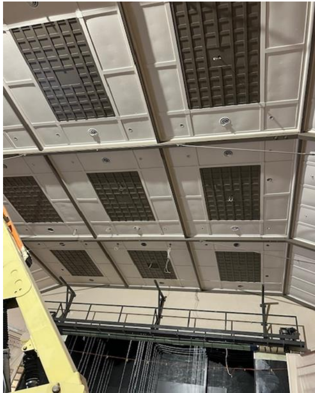
Figure 7 Painting of ceiling complete.
