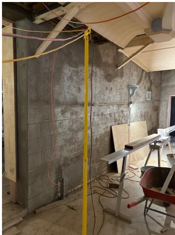
Figure 6 Render to walls to match existing pattern.
