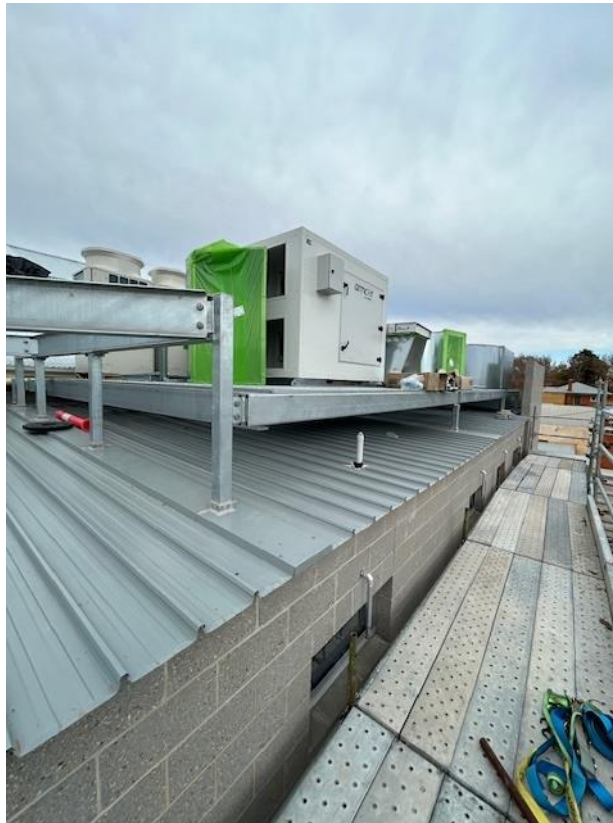
Figure 1 Plant room deck.
