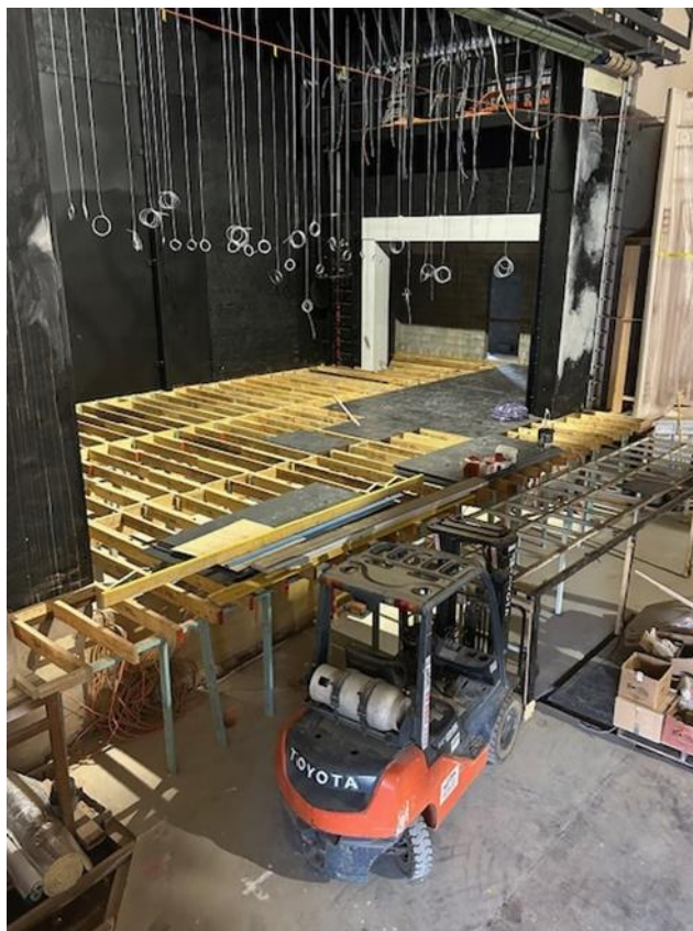
Figure 8 Rebuilt stage and stage rigging.
