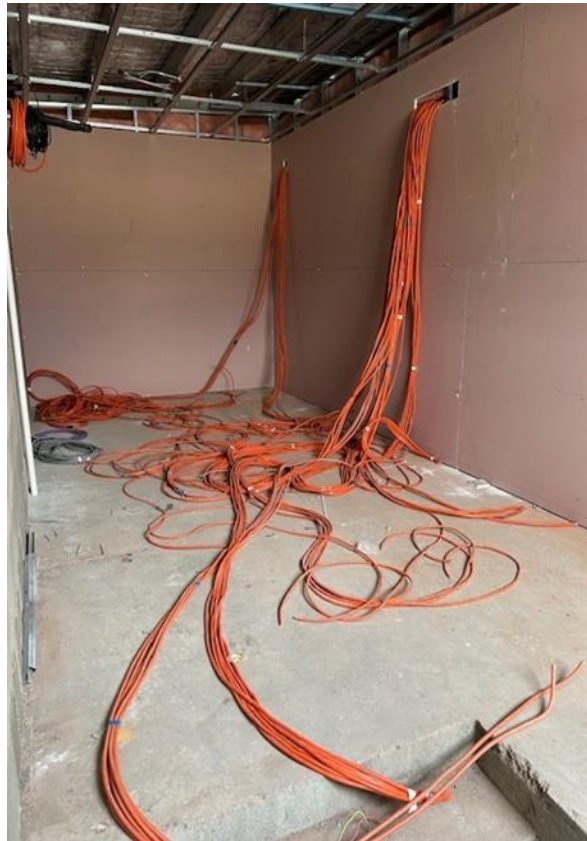
Figure 3 Electrical cable installation.
