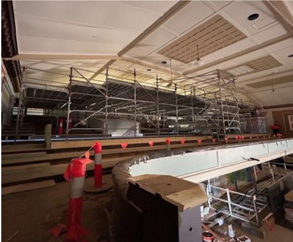
Figure 1 Scaffolding for services and painting - Dress circle.
