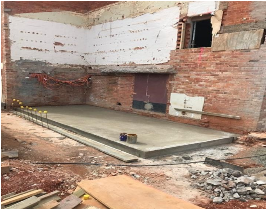
Figure 2 - Southwest external slab for propping
