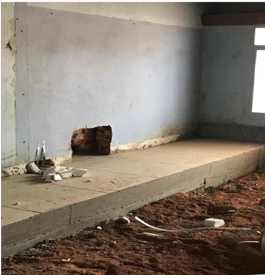
Figure 3 - New edge beam in box office
