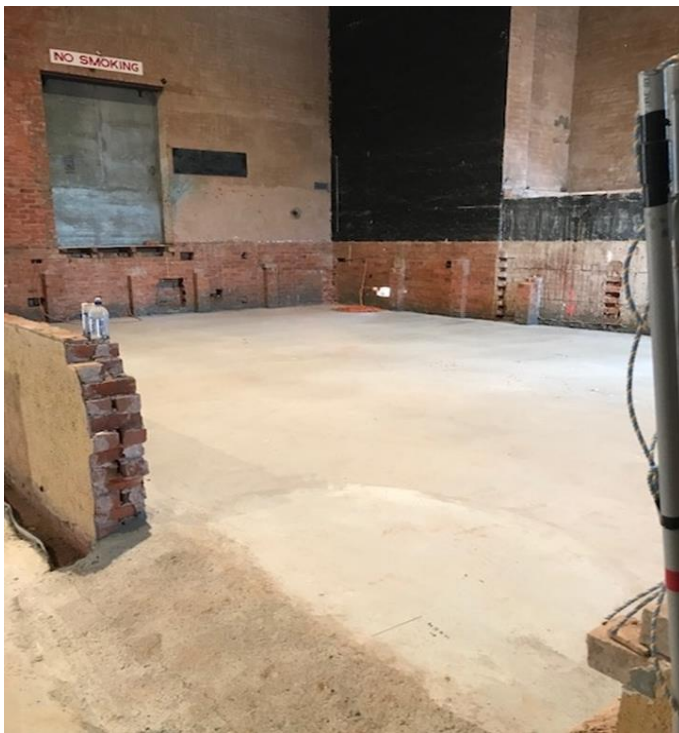
Figure 1 – Sub-stage concrete floor
