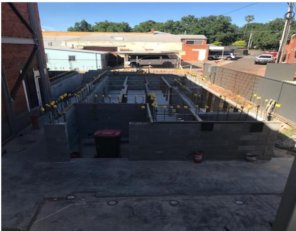
Blockwork rectification and temporary propping for concrete slab
