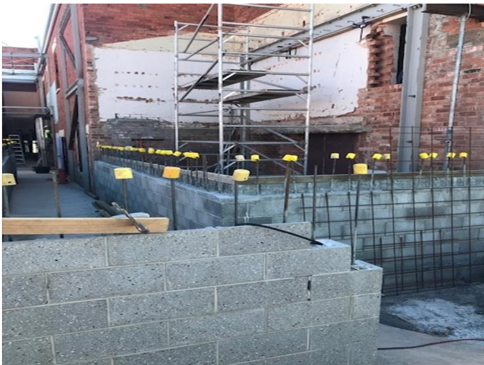
Additional block work -first lift
