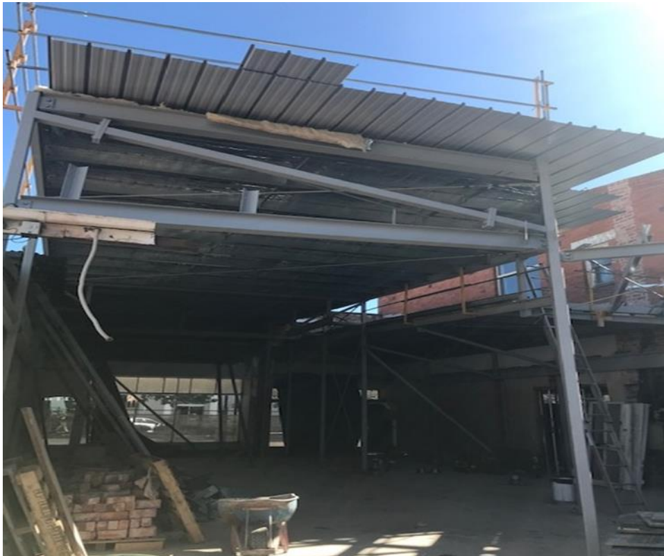
Structural steel in Crate Cafe and new roof
