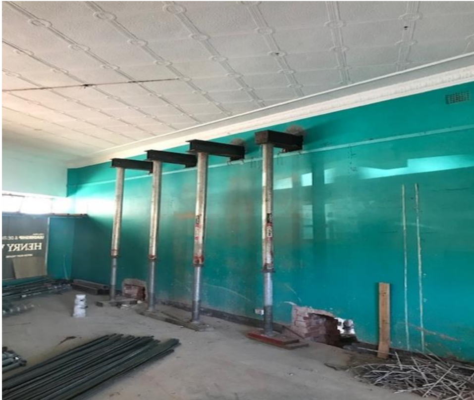
West Wall needle and props
