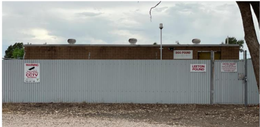
Figure 4 – Subject site (approximate position of new shelter)
