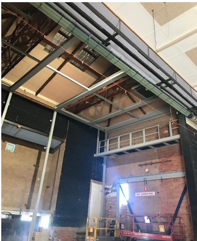
Structural steel to stage
