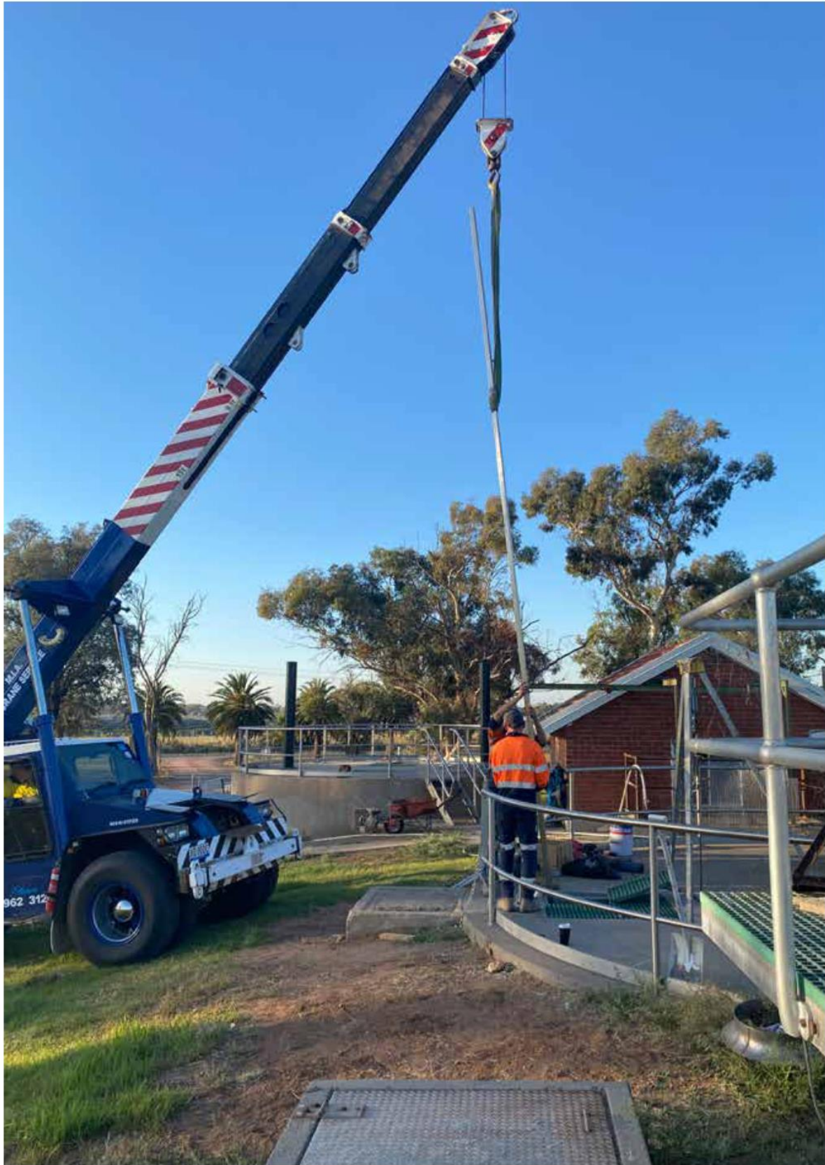
Sewer Plant Upgrade
