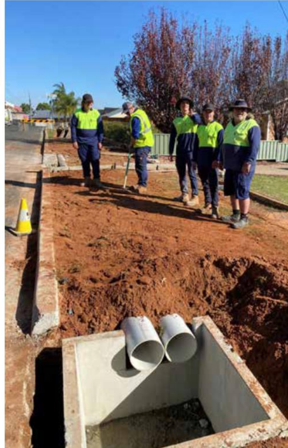
Extending stormwater drainage – Cedar Street
