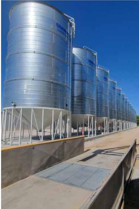
Silo Complex at the Voyager Malthouse, certified and signed off by the Certification Team
