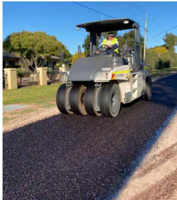
Road sealing works on Almond Road
