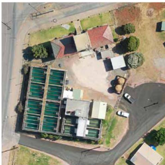
Leeton Water Filtration Plant
