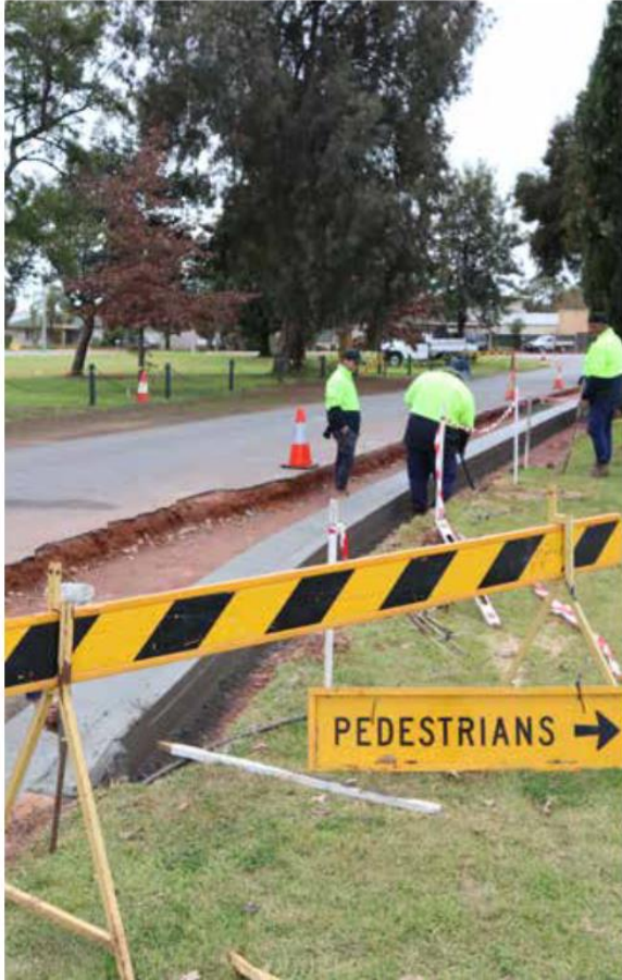
Kerb and guttering Melaleuca Avenue
