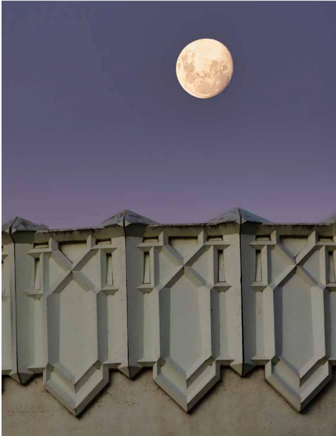
Moonrise over Chelmsford Water Tower Moonrise Photo: Neil McAliece
