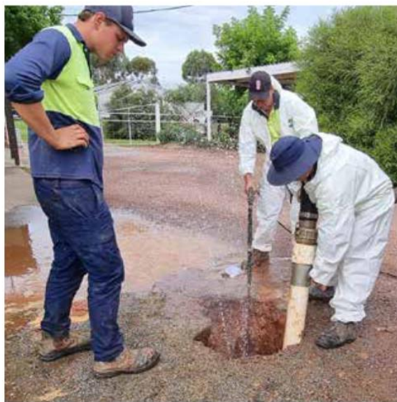
Staff completing repairs on a water main burst
